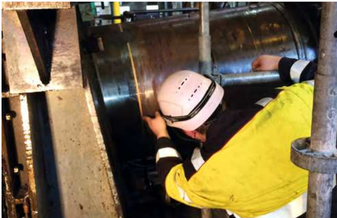
Installation of the telemetry unit
