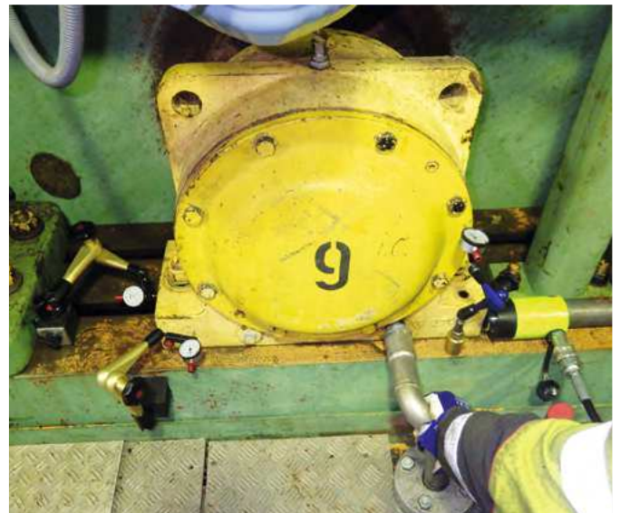
Horizontal roller alignment correction
